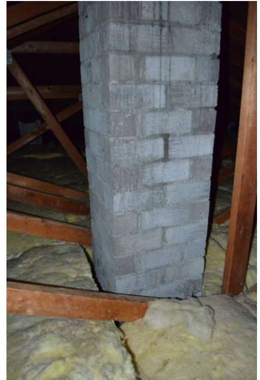
Masonry chimney in an attic.
