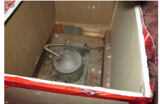
Boxing out existing non-IC-rated pot lights mitigates air leakage at these locations.
