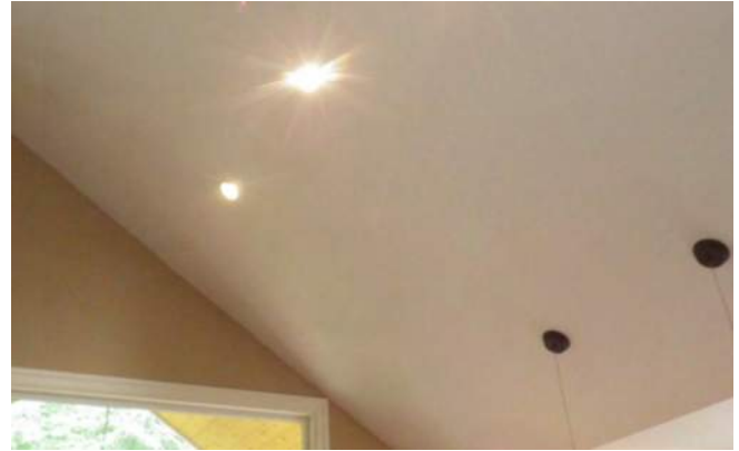
Vaulted gypsum board ceiling with face-mounted and recessed pot light fixtures.
