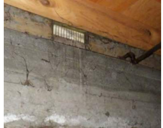
Air vent in the rim joist in an insulated vented crawlspace.
