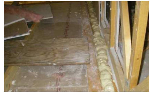
Spray foam installed over top plate joint.
