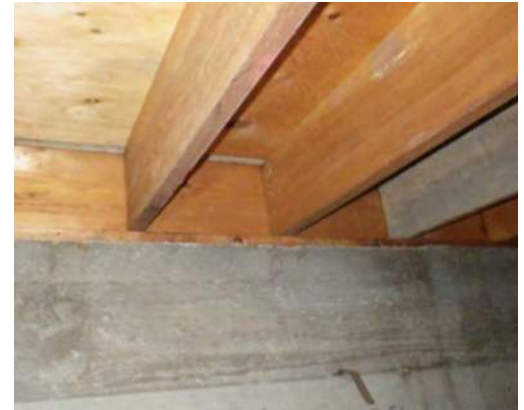
Exposed below-grade wall at floor rim joist.
