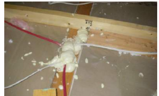
Top plate penetrations sealed with spray foam.
