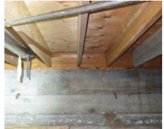
Uninsulated crawlspace interior walls and floor.
