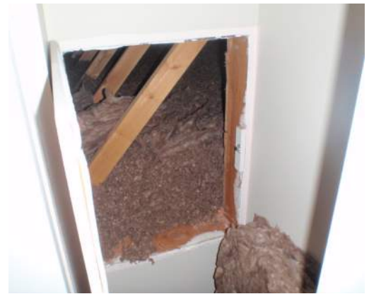
Access hatch at knee wall.
