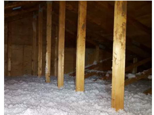
Gable end wall.
