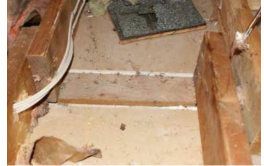
Exposed interior top plate as viewed from the attic.
