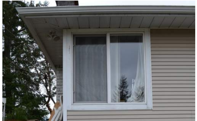
A window located on a facade with low rain exposure, protected by a large overhang.
