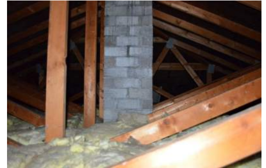
Accessible attic with trusses, batt insulation, and a masonry chimney.
