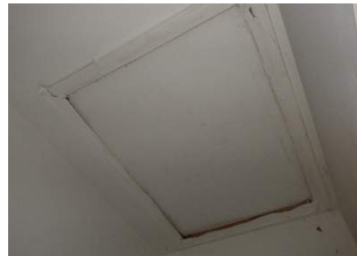
An attic access cover made from plywood resting on a wood-trimmed opening.
